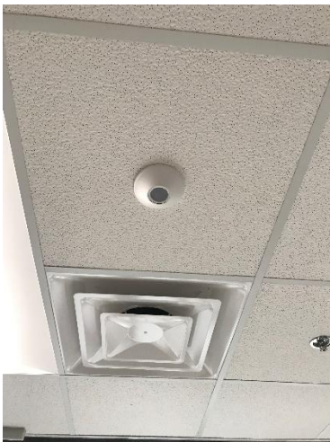
Image of a typical ceiling mounted occupancy sensor
