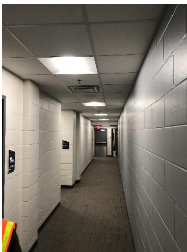
Image of a typical corridor lighting
