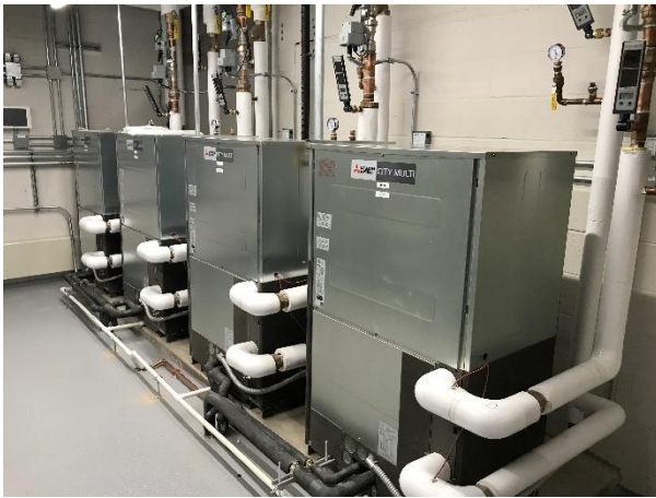
Image of typical water source heat pumps
