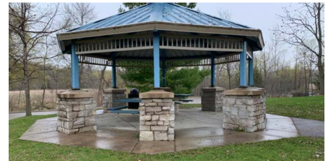
Picnic shelter at Meadow Park
