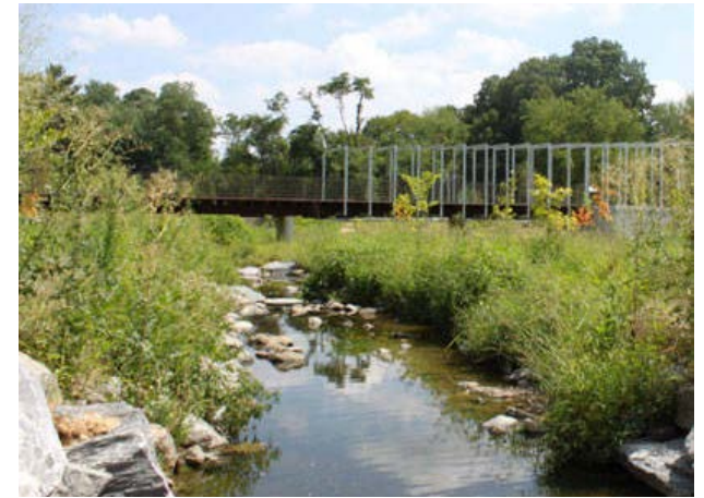
Example of incorporating stormwater best practices
