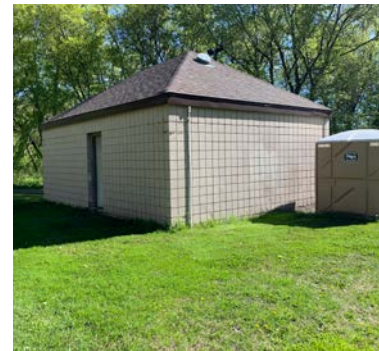
Warming house and restroom at Covington Park
