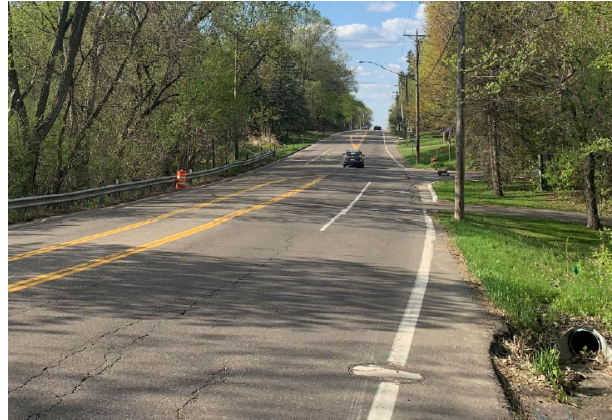
Existing conditions – Hopkins Crossroad (looking north)
