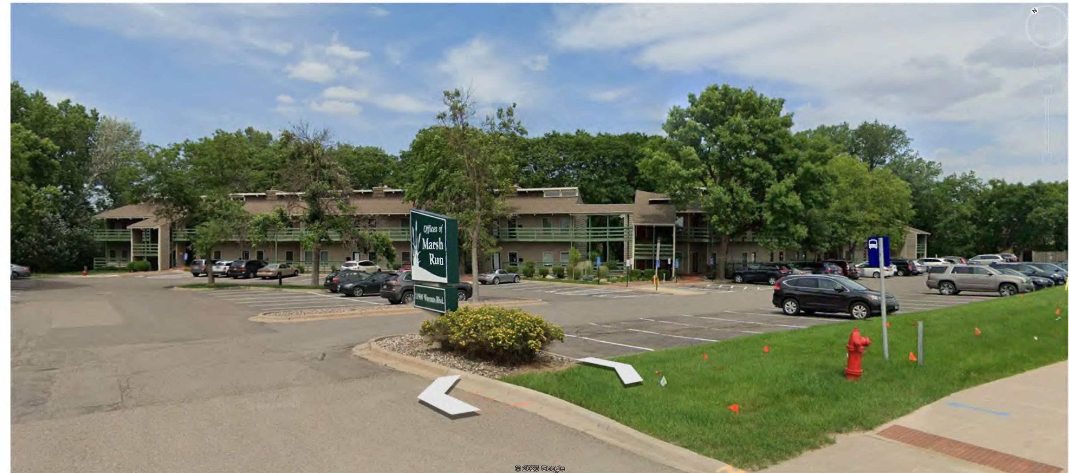
STREET VIEW FROM SW CORNER
