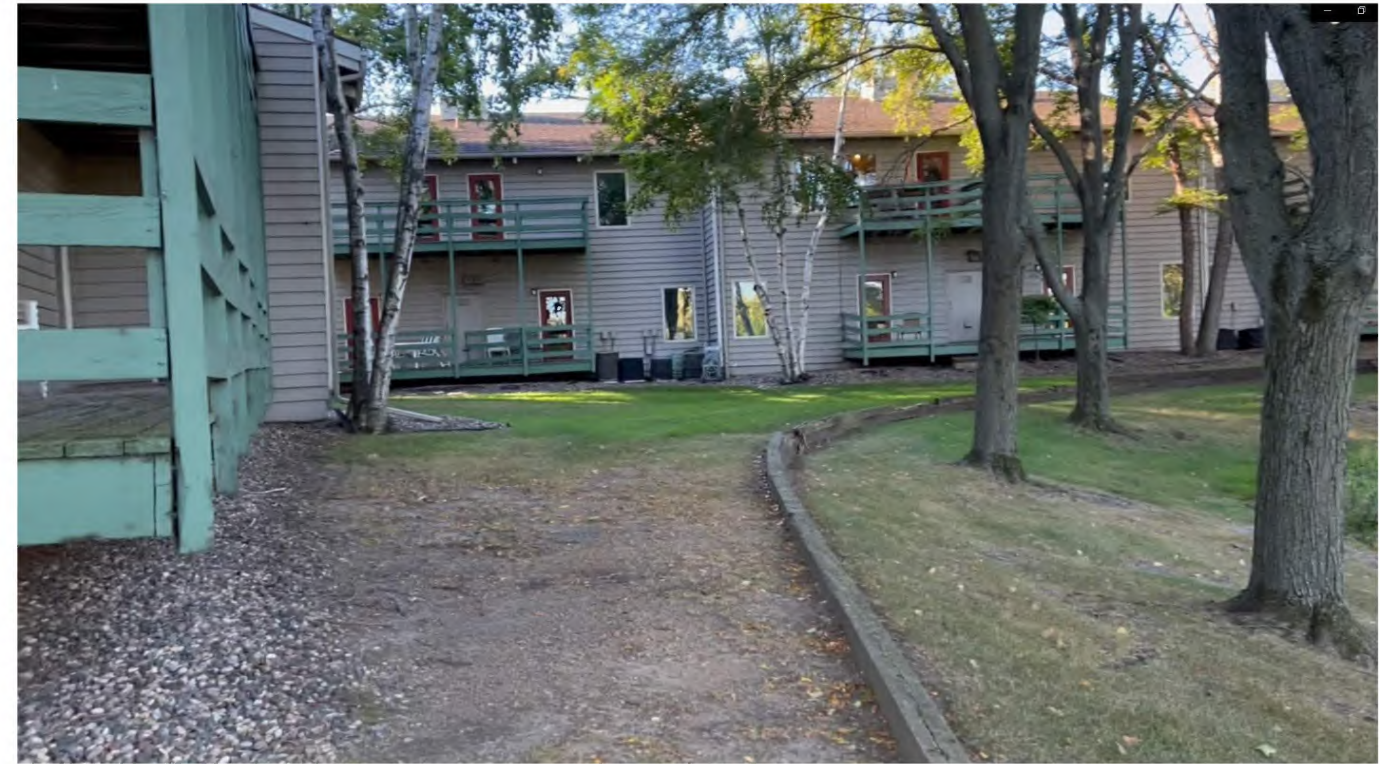
VIEW FROM NE CORNER
