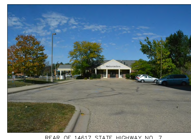
REAR OF 14617 STATE HIGHWAY NO. 7 CITY OF MINNETONKA, HENNEPIN COUNTY, MINNESOTA
