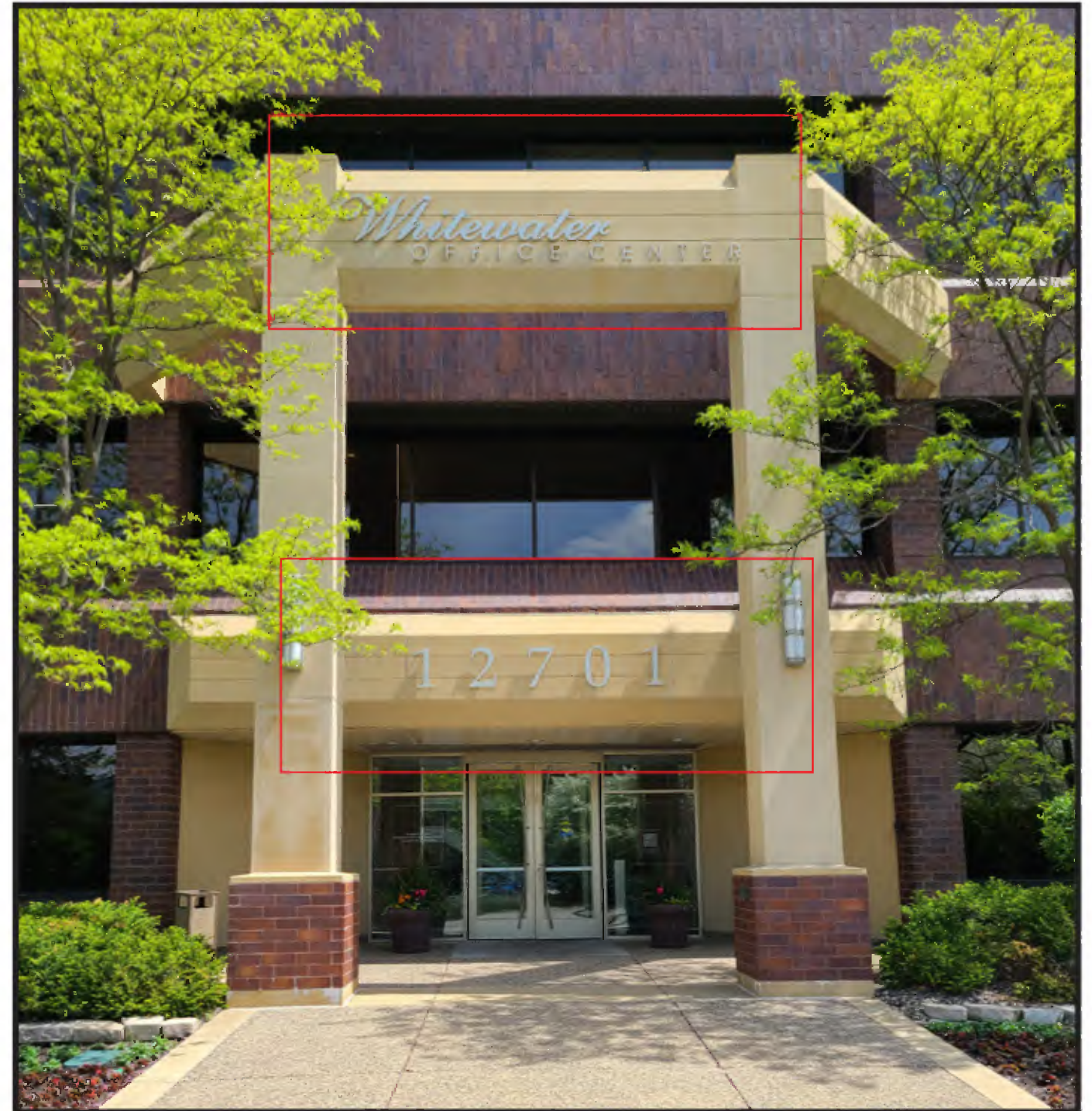
Existing 12701 Entrance to be Removed
