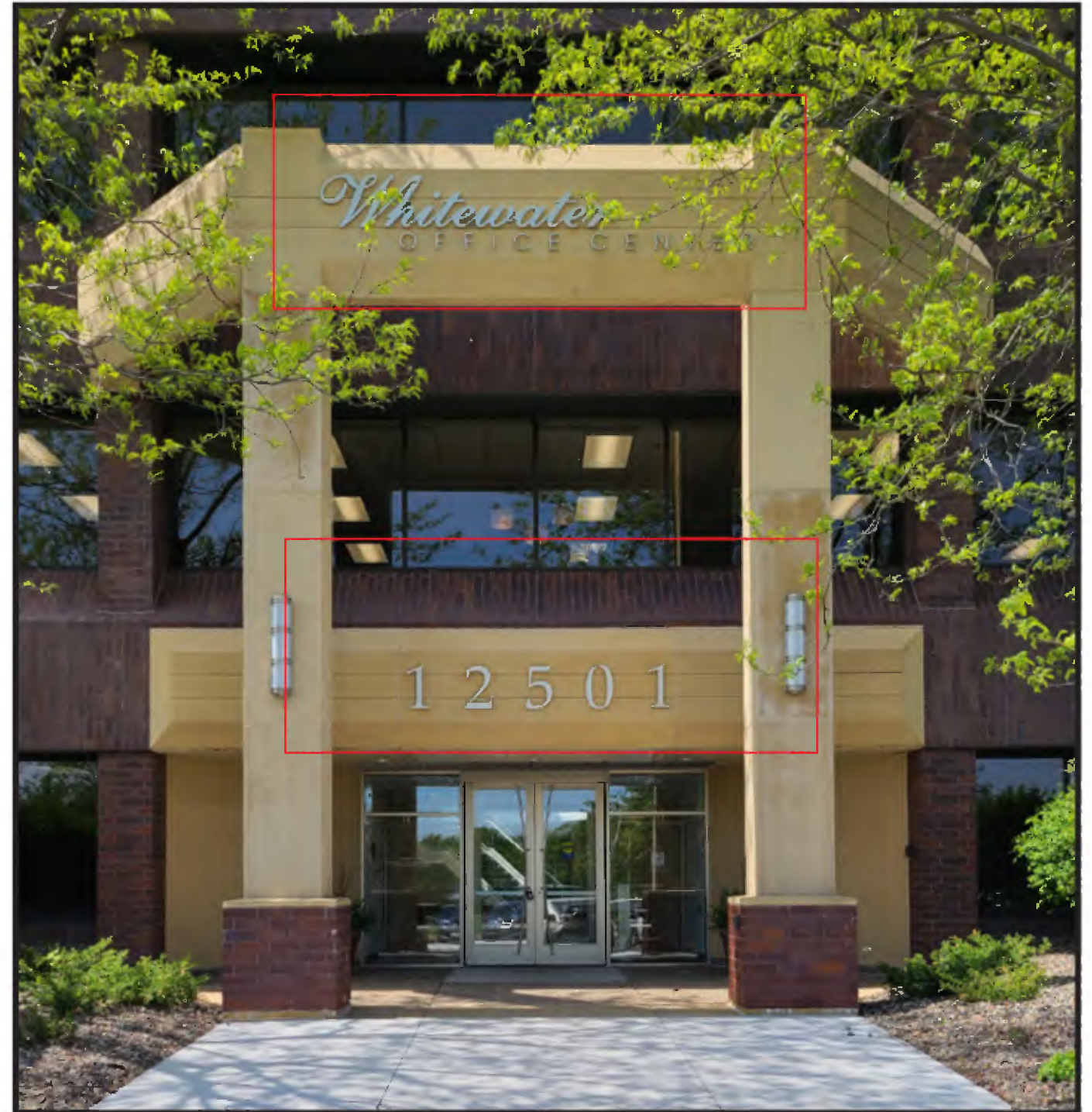
Existing 12501 Entrance to be Removed
