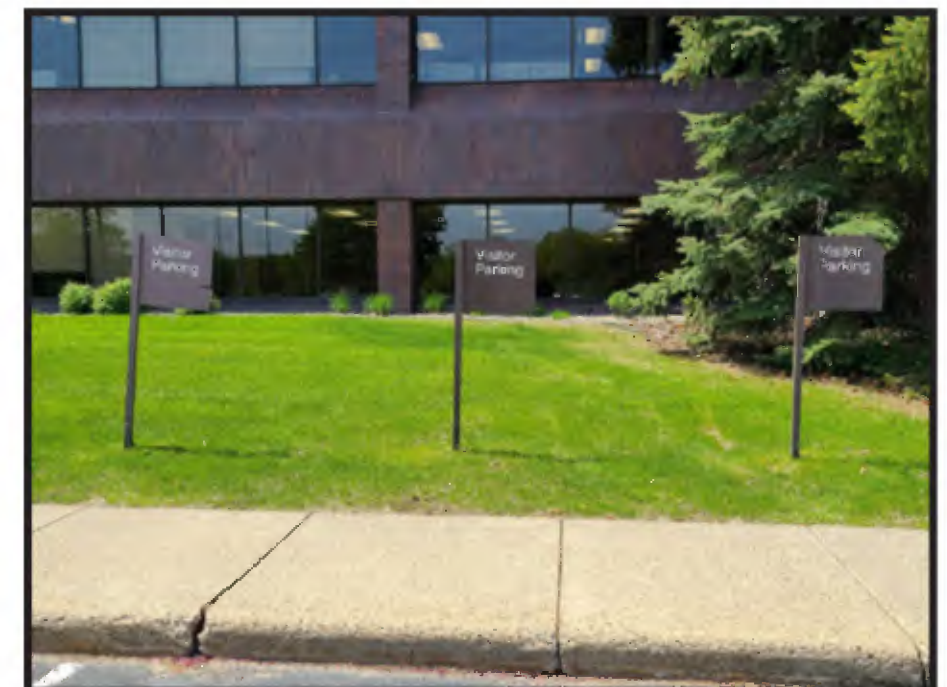
(6) Existing Visitor Parking Signs to be Removed
