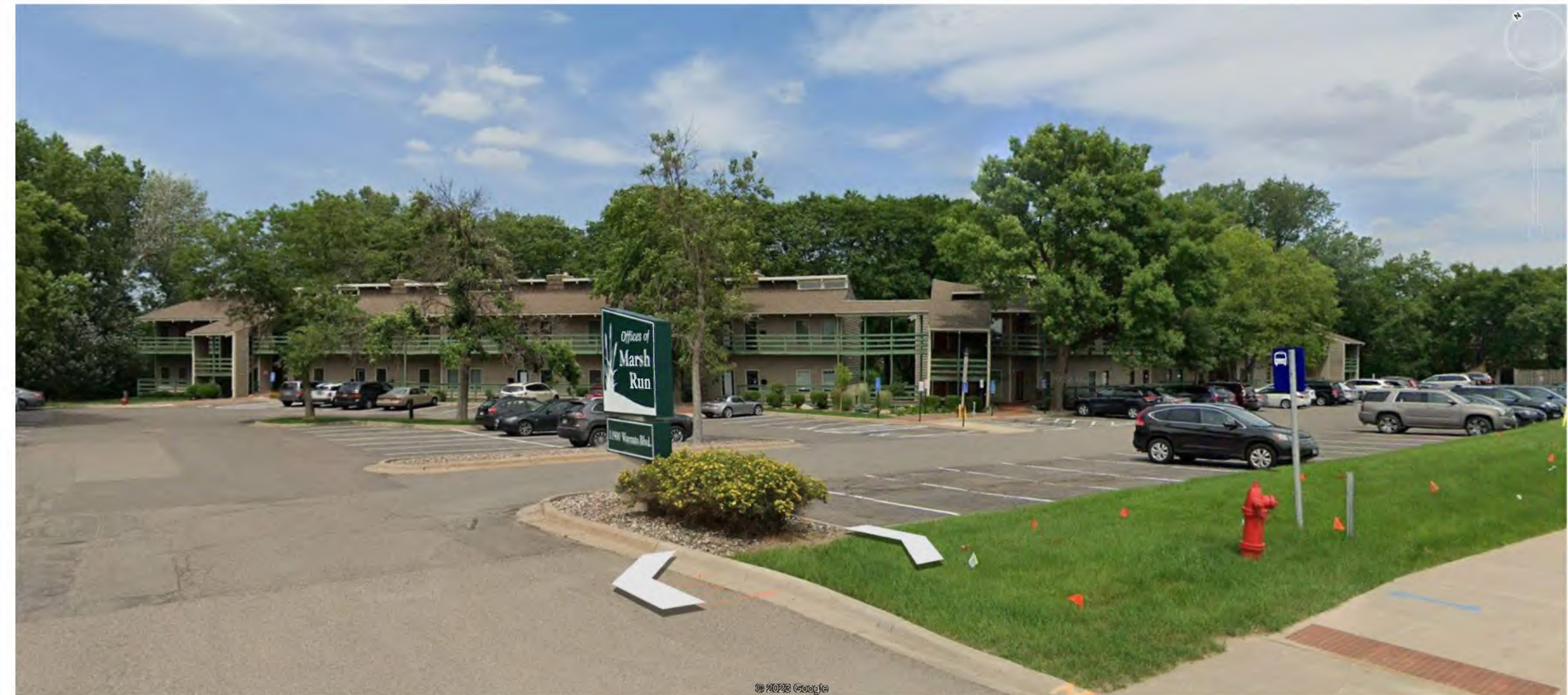
STREET VIEW FROM SW CORNER
