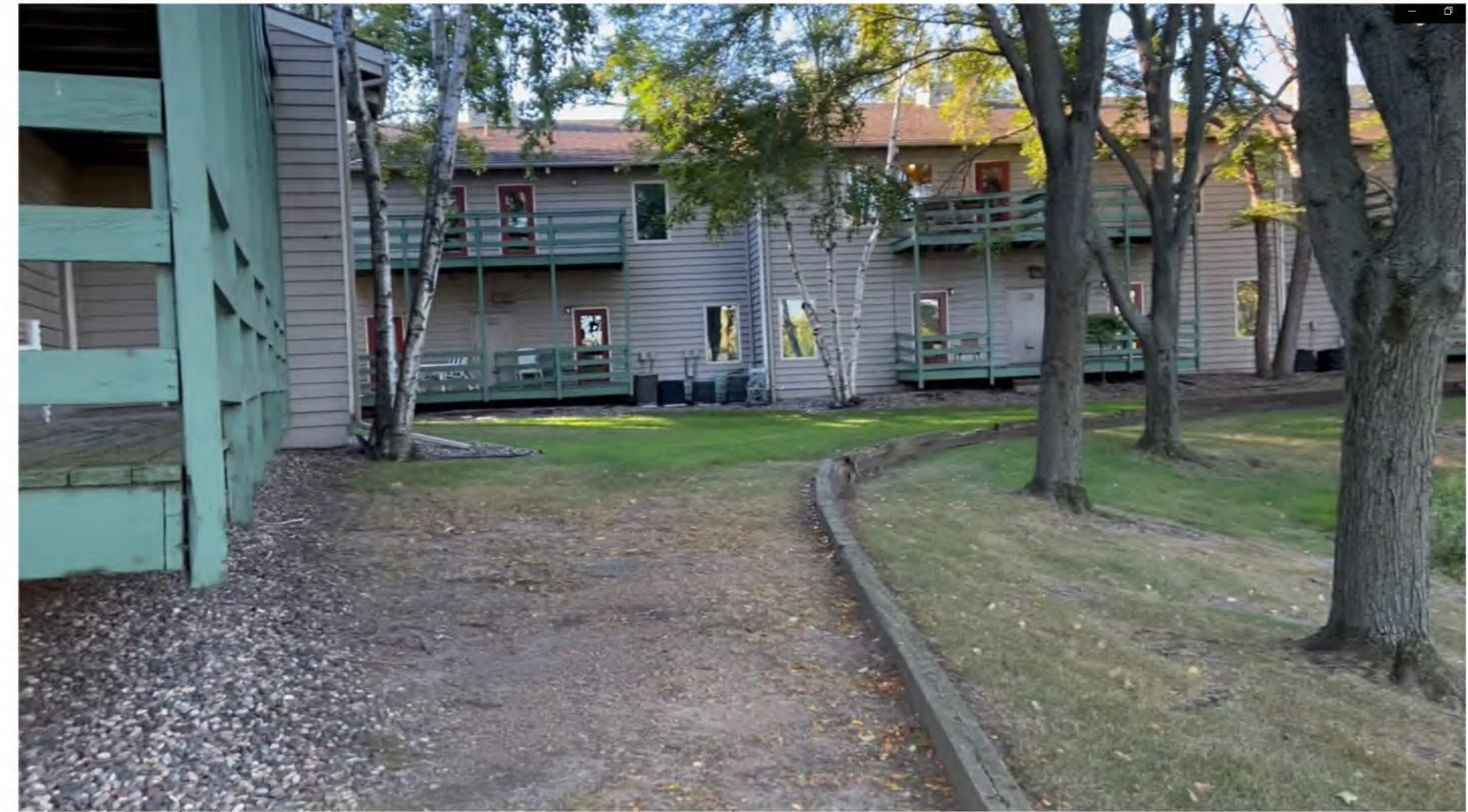
VIEW FROM NE CORNER
