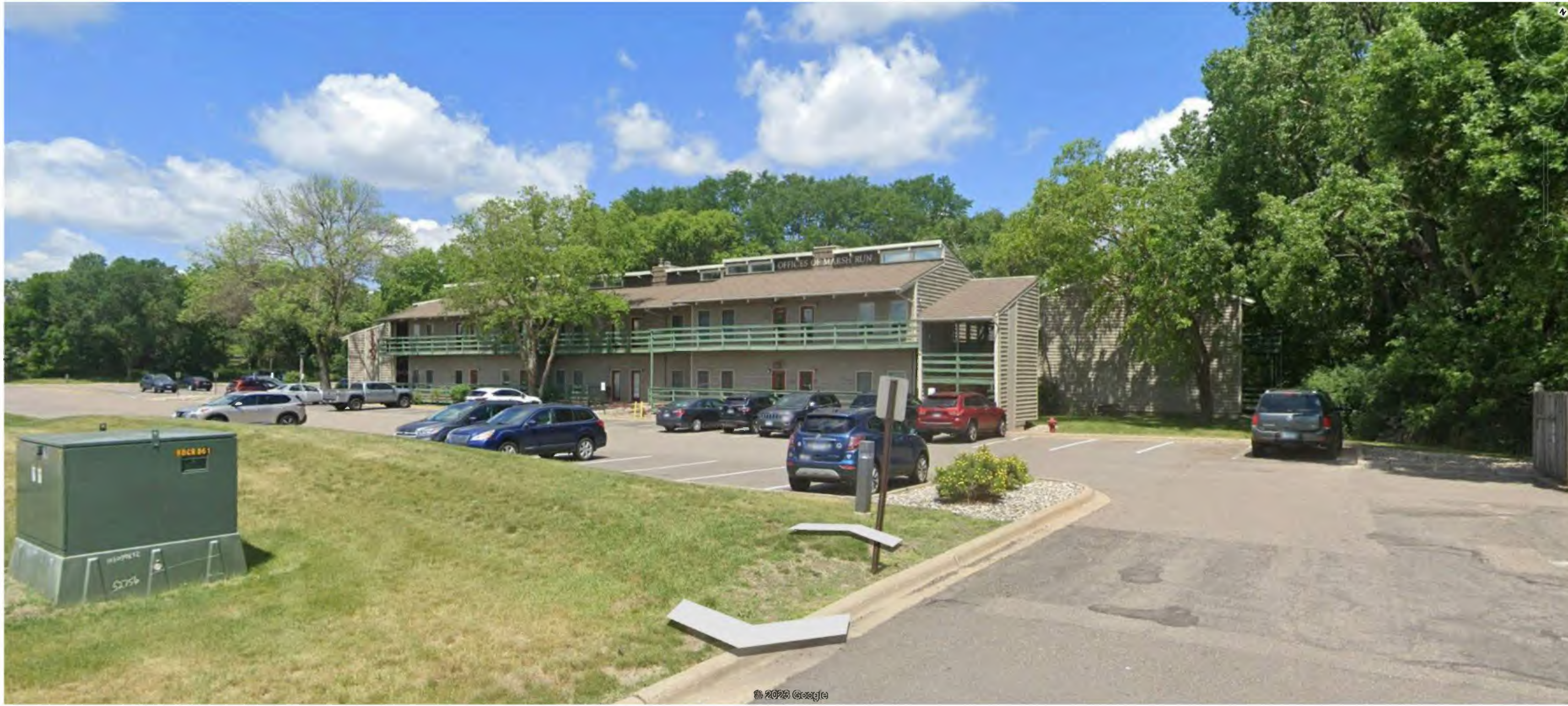
STREET VIEW FROM SE CORNER
