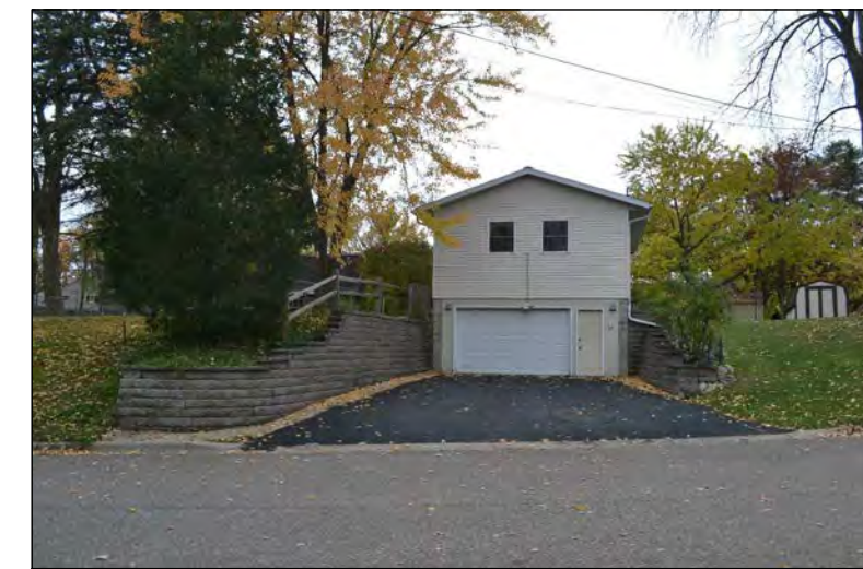
FRONT OF GARAGE AT 13910 KNOLLWAY DRIVE SOUTH CITY OF MINNETONKA, HENNEPIN COUNTY, MINNESOTA
