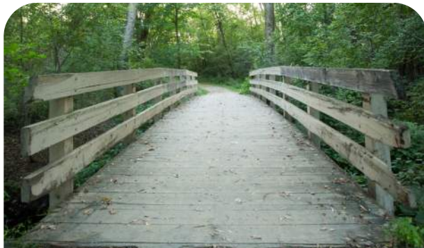
Timber bridge near main parking lot
