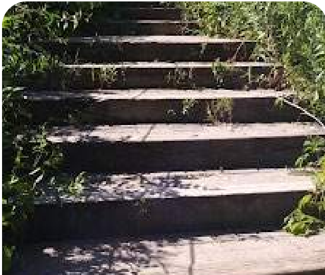
Example of timber stairs with paver treads
