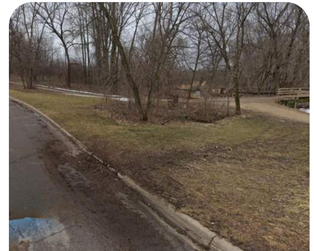
Existing drainage issues along main entrance road adversely affecting nearby trails, vegetation and curbs
