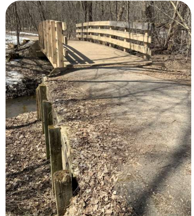
Timber pedestrian bridge near main parking lot
