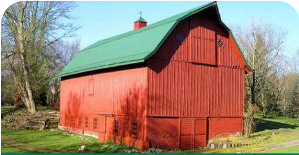
Existing Red Barn structure
