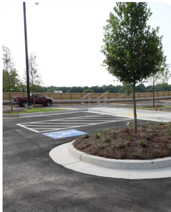
Bituminous surfacing with curb + gutter
