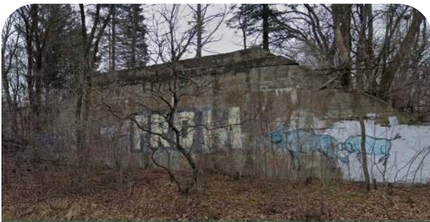
Existing bridge abutment
