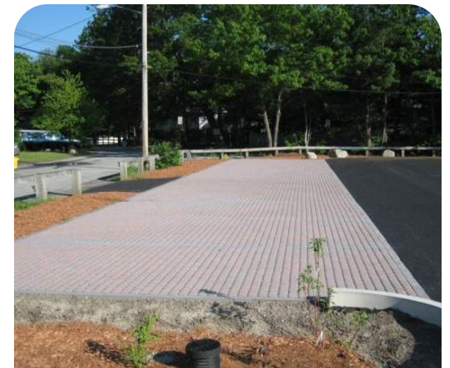
Bituminous drive w/ permeable paver parking
