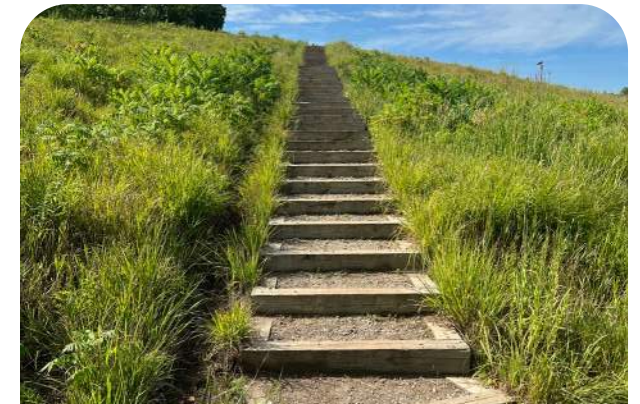
Timber stairs on east side of park
