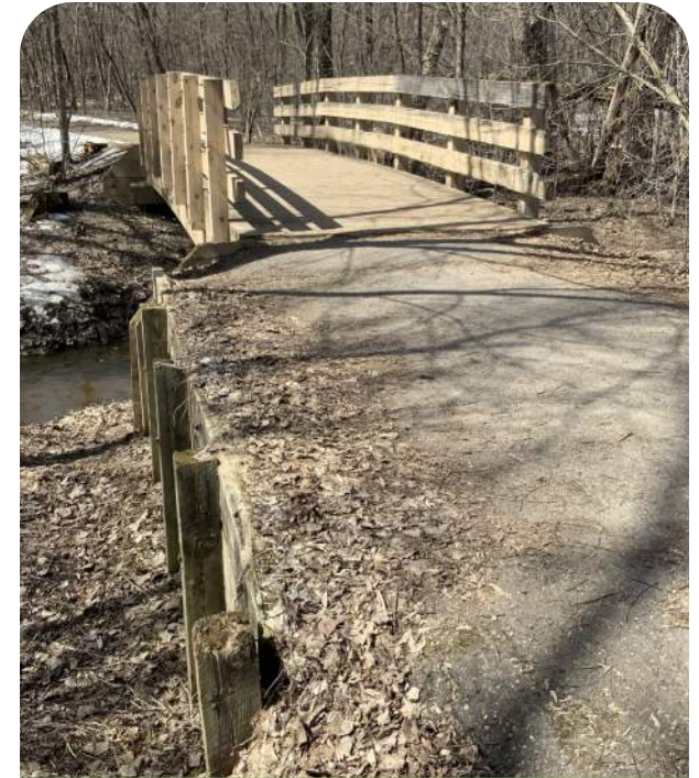
Timber pedestrian bridge near main parking lot
