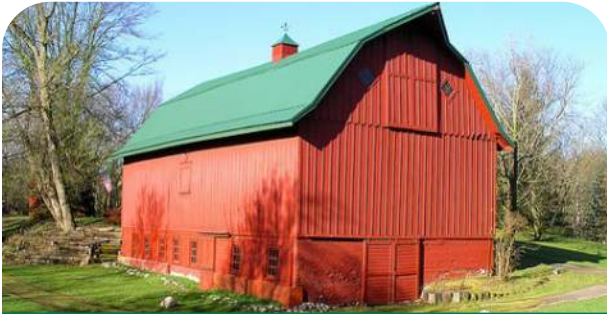
Existing Red Barn structure
