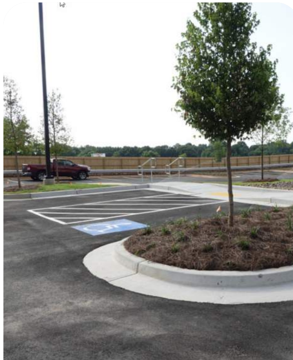
Bituminous surfacing with curb + gutter
