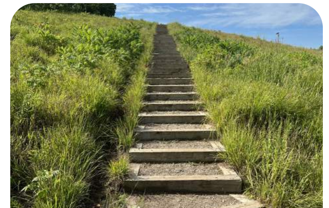
Timber stairs on east side of park
