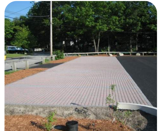
Bituminous drive w/ permeable paver parking
