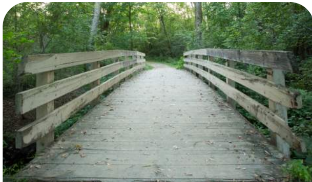
Timber bridge near main parking lot
