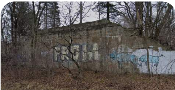
Existing bridge abutment
