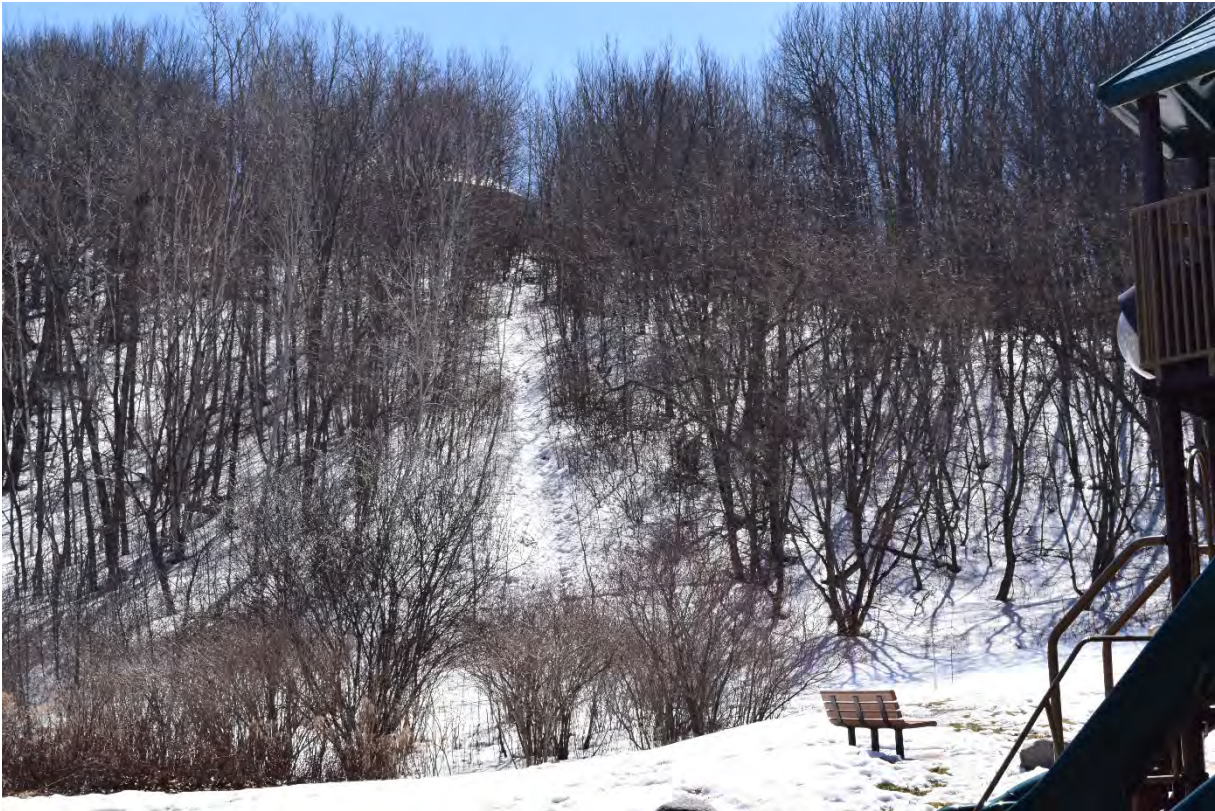
Vertical trail from water tower to playground, with sever erosion.
