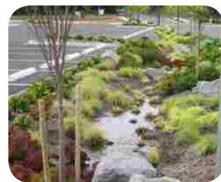
Fig. 69: Bioswale incorporated into parking lot
