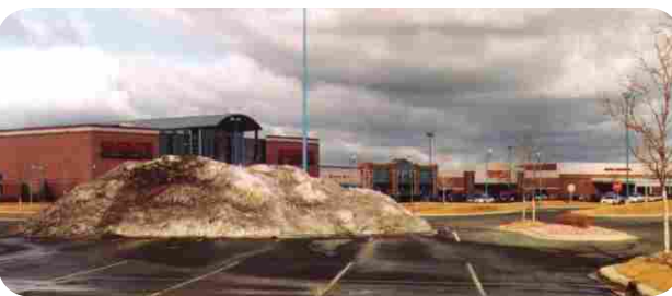
Fig. 70: Snow plowed and piled in parking lot. Consideration should be given to locating these “snow dumps”, since they will contribute a significant amount of stormwater runoff.
