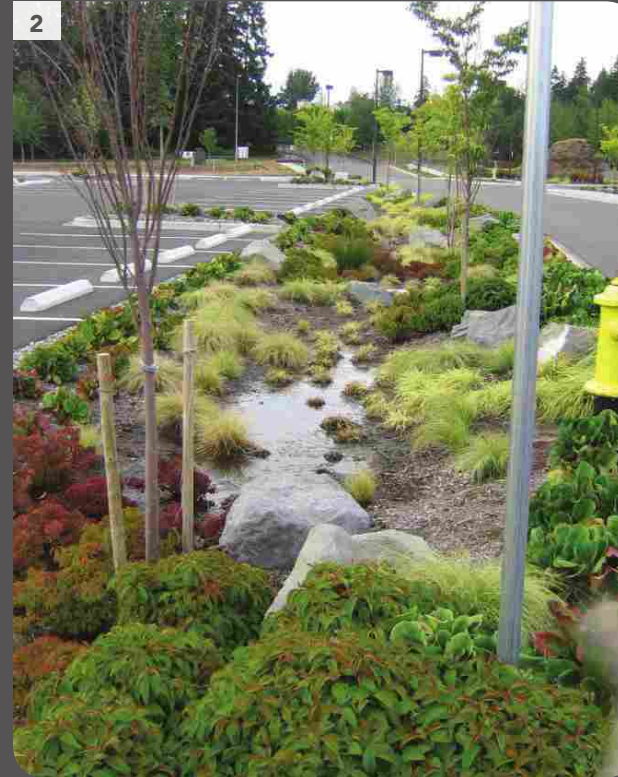
1. Bioswale along pedestrian trail 2. Bioswale in parking lot median
