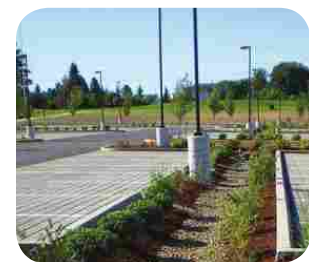
Fig. 64: Use light-colored, permeable paving
