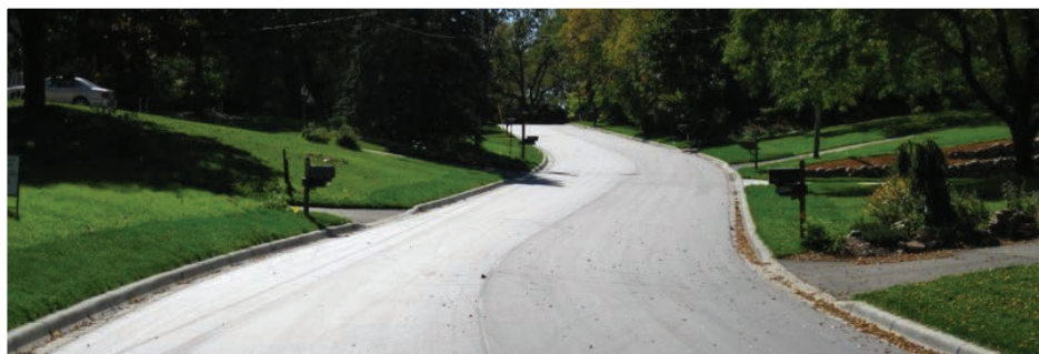
After street reconstruction
