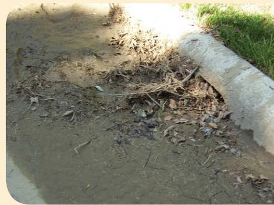
One easy way to protect water quality – be sure storm drains are clear of debris.
