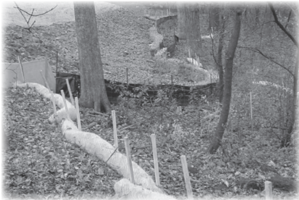
This photo shows several erosion control techniques.
