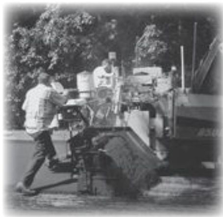
Crews install thin overlay on a street.
