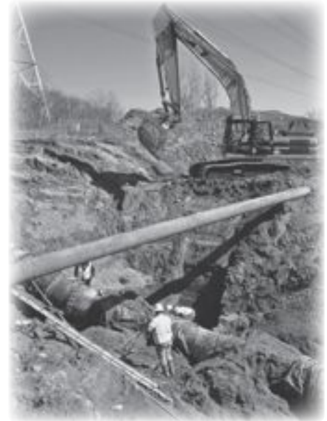
Water main work at Orchard Road
