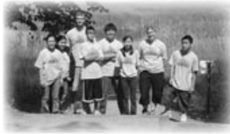
Tree Trust youth stand at the top of the stairs they built at the Jidana Park canoe landing.
