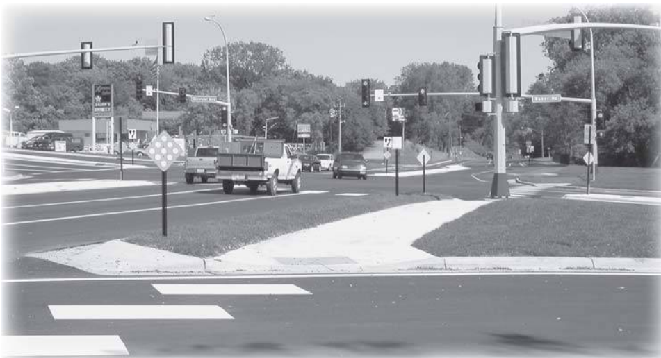
The reconstructed intersection at Baker Road and Excelsior Boulevard opened in September.
