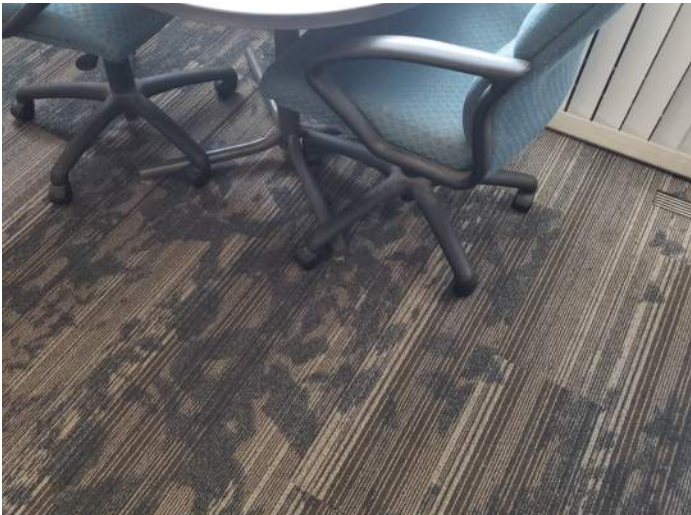
FIGURE 18: New carpet finish in private offices; approximately one year old.
