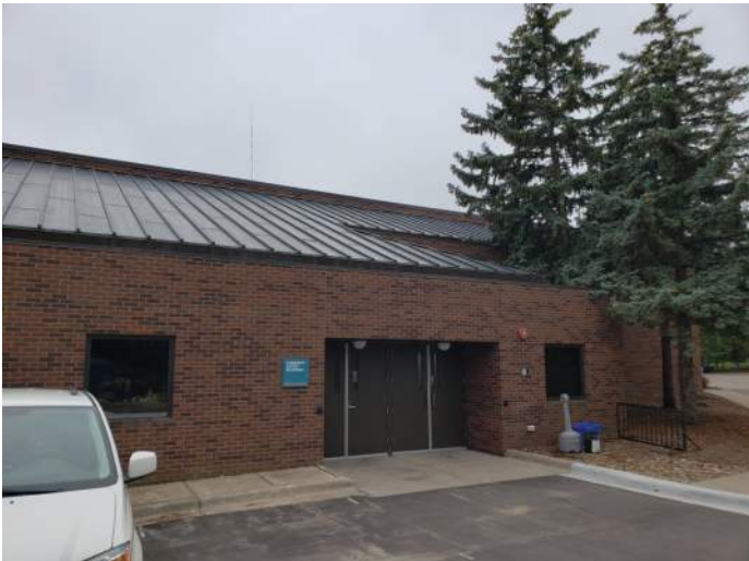
FIGURE 2: Standing seam copper roof is in good condition.
