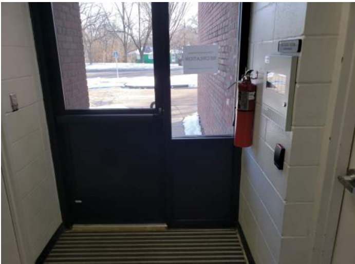
FIGURE 12: Aluminum entrances are in good condition.
