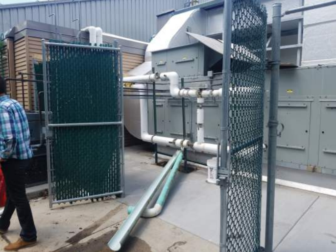
FIGURE 41: Pool dehumidification unit is in the process of being replaced.
