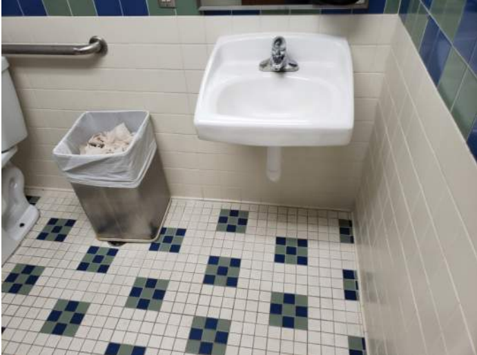
FIGURE 16: Accessible wall-hung lavatory in good condition.
