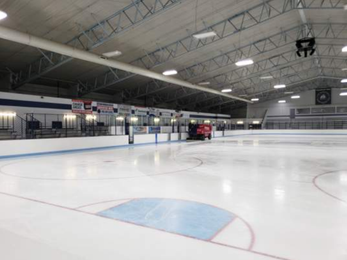
FIGURE 22: Arena A - new boards installed within last year.
