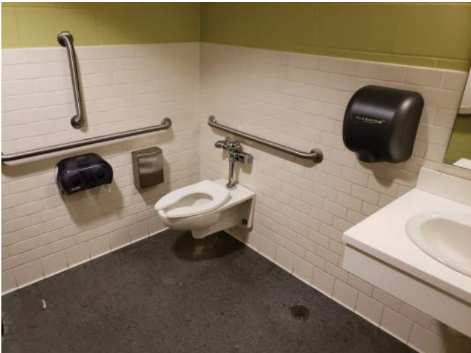
FIGURE 20: Lower level restrooms are in good condition and accessible.
