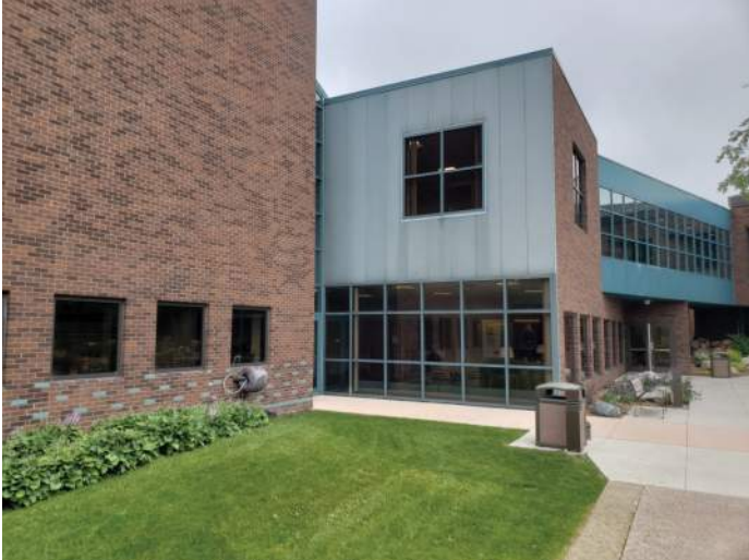
FIGURE 13: Metal panels are faded and discolored. Recommend repainting metal panels to improve appearance.
