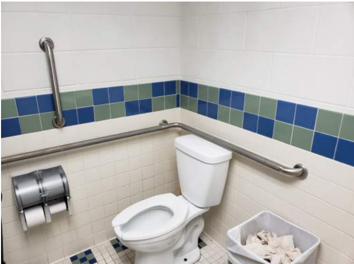
FIGURE 17: Accessible watercloset in good condition.
