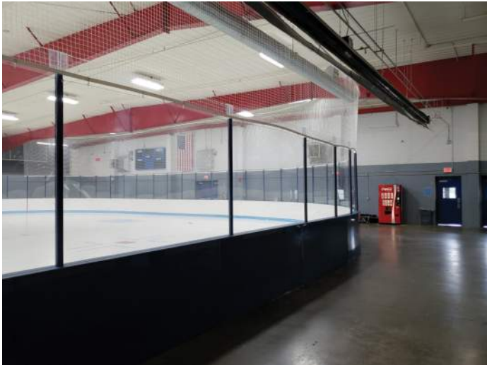
FIGURE 36: New boards installed in Arena B within last year.
