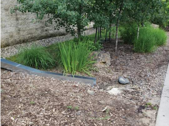
FIGURE 4: Downspout is eroding landscape. Recommend adding rock or other materials to prevent erosion.
