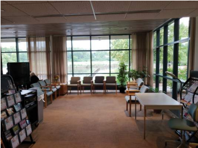
FIGURE 33: Worn, aged carpet and ceiling tiles in Glen Lake Room. Recommend replacing carpet and ceiling tiles.
