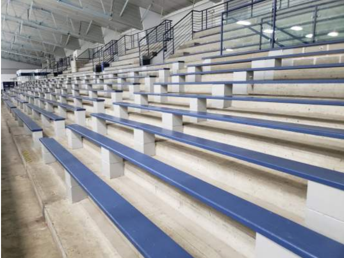
FIGURE 25: Bench seating and railings are in good condition.
