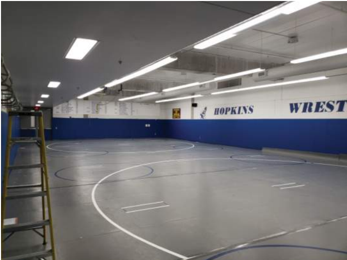
FIGURE 12: Wrestling room - finishes observed were in good condition.
