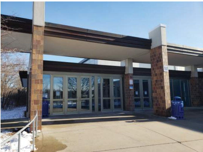
FIGURE 23: Aluminum framed entrance system was observed to be in good condition.
