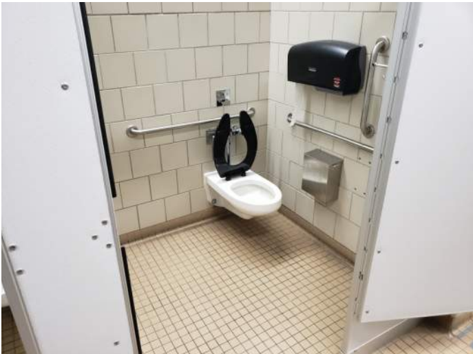
FIGURE 14: Accessible toilet stall.
