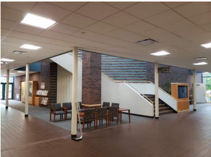
FIGURE 24: Interior finishes in lobby space are overall in good condition.
