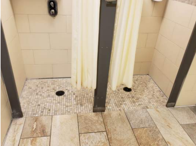
FIGURE 31: Showers in locker rooms are newly tiled and in good condition.
