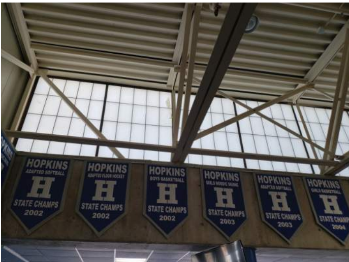
FIGURE 20: Translucent panels were observed to be in good condition.
