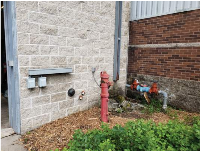
FIGURE 15: Downspout empties directly at building wall, recommend installing downspout extensions to direct water away from building.
