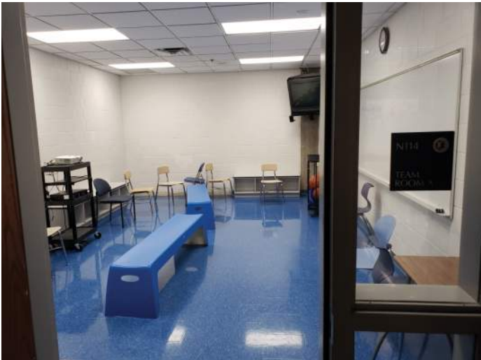
FIGURE 15: Team room - finishes observed were in good condition.
