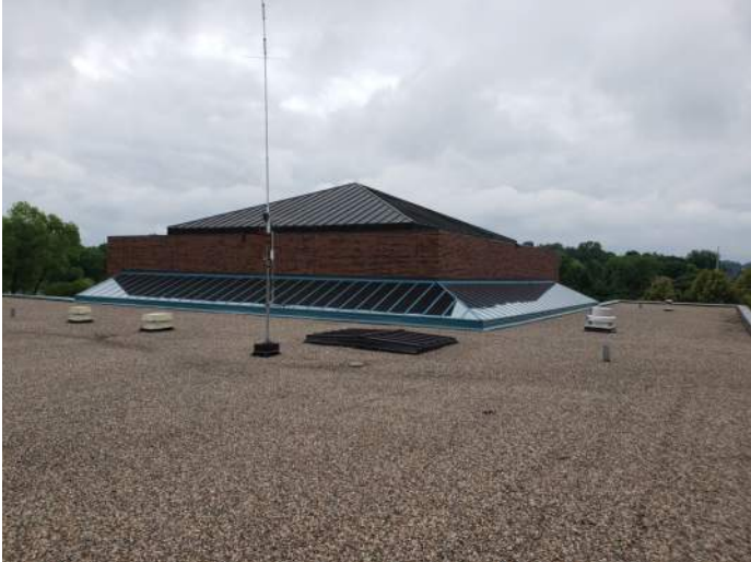
FIGURE 19: Roof area appears to be in good condition.
