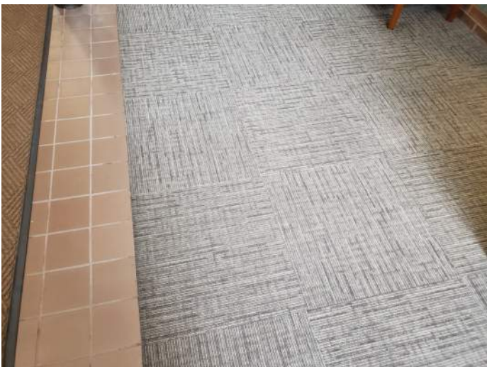
FIGURE 27: New carpet installed in lobby in 2018, like-new condition.
