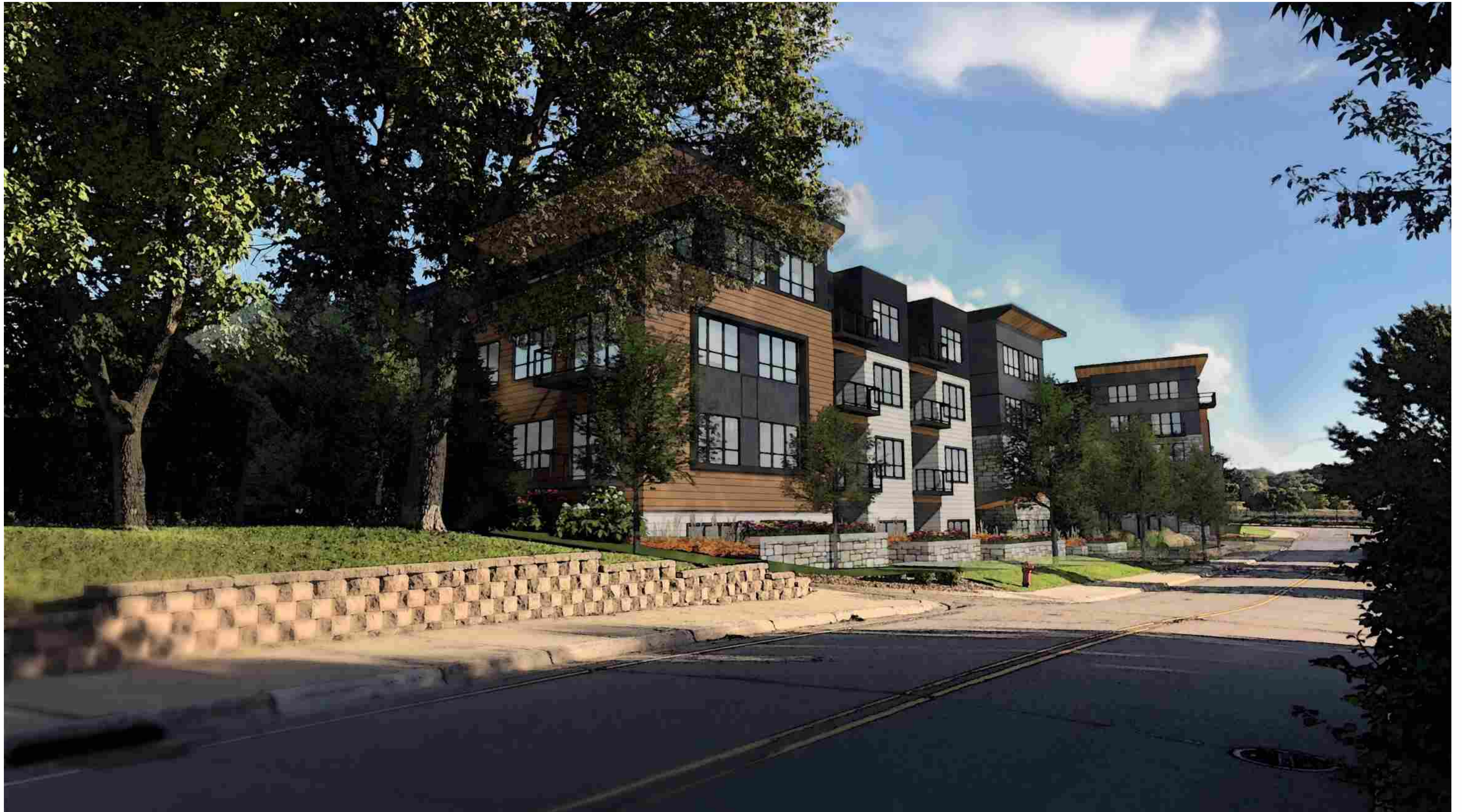
LOOKING SOUTH ON FAIRFIELD AVE.
