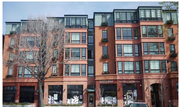
The developer of this 38-unit property in Berkeley, California, provided seven affordable units in exchange for an extra story.
