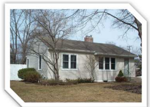
Home after renovation:
