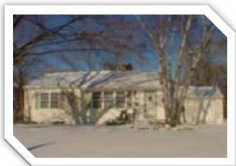
Home prior to renovation
