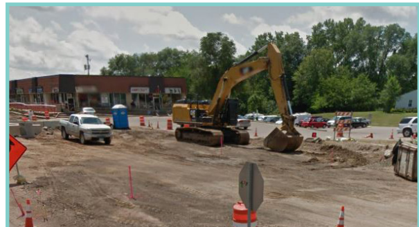
Shady Oak Road Reconstruction - facing 4312 Shady Oak Road
