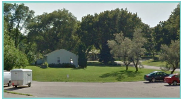
Shady Oak Road Reconstruction - facing 4292 Oak Drive Lane
