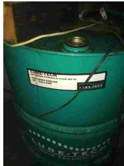
Photo 8: Hydraulic oil stored in the Mid-Tool space.
