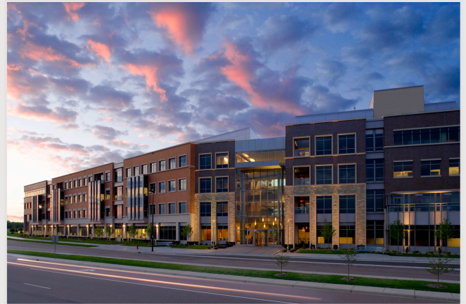
Office development that fronts the street
