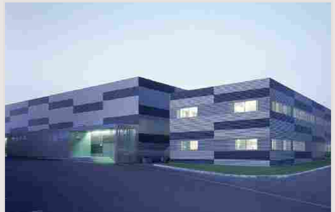
Shielded loaded bays to the rear of the building
