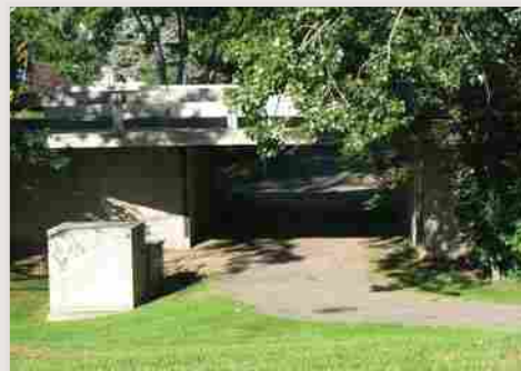
Existing trail underpass
