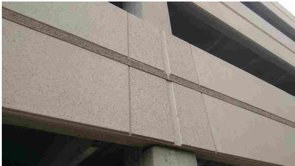
Detail of acid washed panels with exposed aggregate accent stripe
