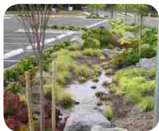
Fig. 69: Bioswale incorporated into parking lot
