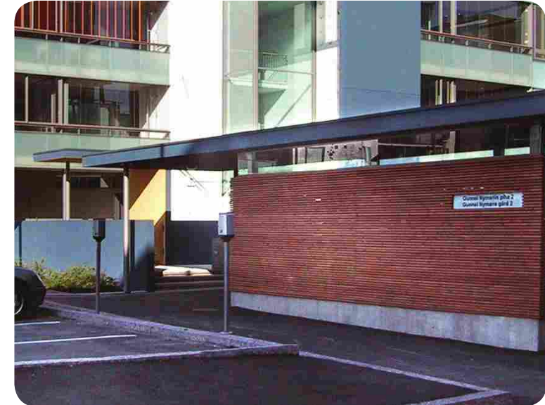
Fig. 72: Design Checklist 2: Trash areas are screened from view and do not negatively impact on the appearance of the building or street
