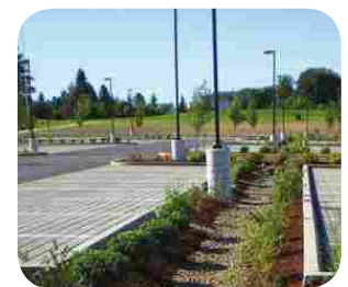
Fig. 64: Use light-colored, permeable paving
