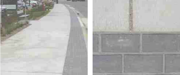
Fig. 41: Typical Concrete Sidewalk with Brick Warning Strip - 1700 Plymouth (Catalyst Project for Ridgedale Area)
