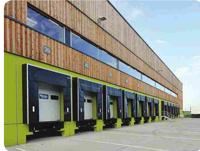
Fig. 71: Design Checklist 1: Loading and servicing is provided for and does not interrupt or interfere with vehicle or pedestrian access
