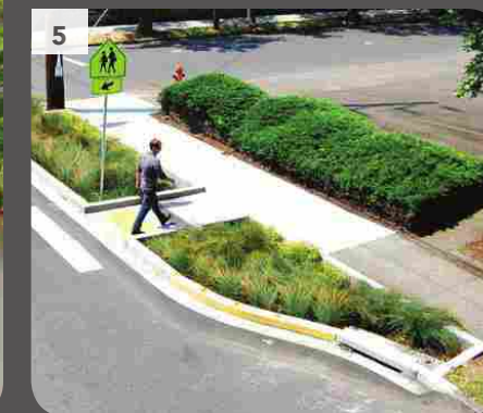
3. Rain garden adjacent to surface parking lot and sidewalk 4. Permeable Paving 5. Bioswale between sidewalk and roadway
