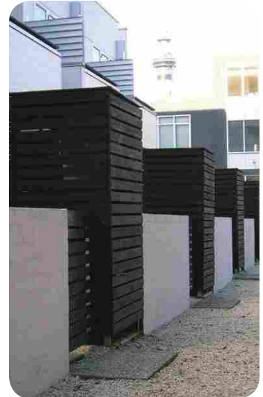
Fig. 73: Design Checklist 3: Refuse and recycling stations are provided in convenient yet discrete locations (Beaumont Quarter, Auckland)
