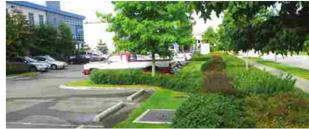
Fig. 74: Bioswale continuous along roadway
