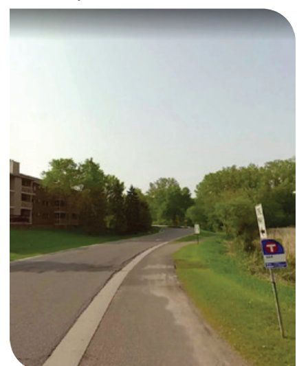
Bus stop sign without shelter, bench or sidewalk.
