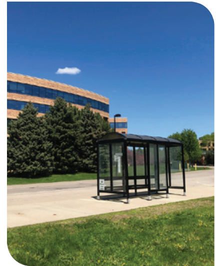
Bus stop with shelter and sidewalk.
