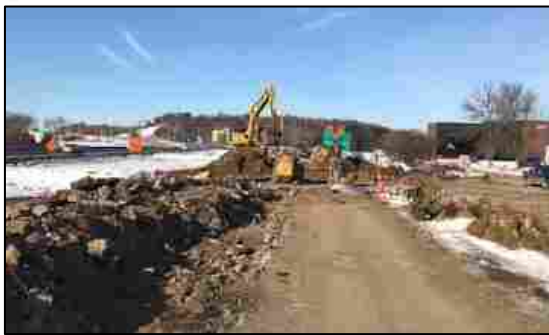
Excavation for Hwy 62 LRT Tunnel
