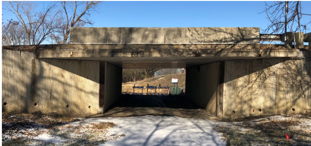
Existing bridge at Bren Road West
