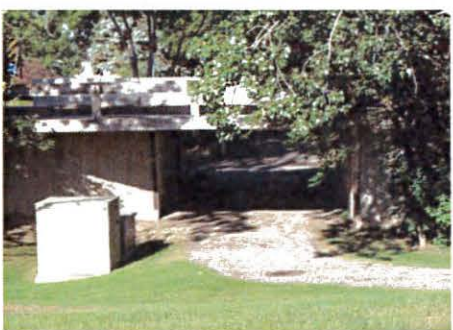
Existing trail underpass
