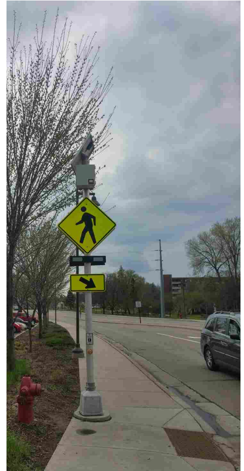
Pedestrian crossing improvement at Woodhill Road and Excelsior Boulevard
