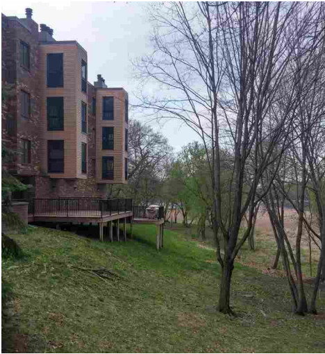
Looking south into the East (South) Site
