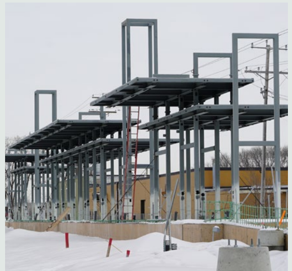
Shady Oak Station construction
