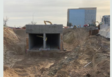
Hwy 62 tunnel construction
