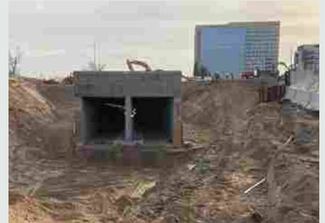
Hwy 62 tunnel construction
