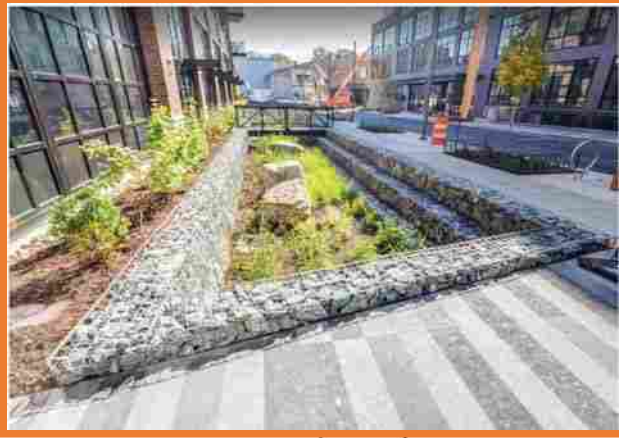
STORMWATER LANDSCAPE ELEMENT
