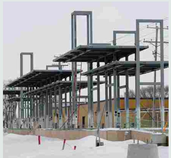
Shady Oak Station construction
