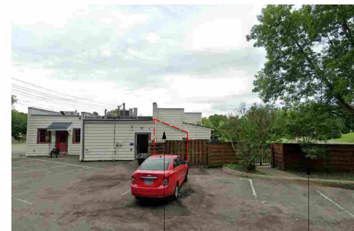
REMOVE EXIST OUTDOOR STORAGE LEAN-TO (6'-4" x 9'-4") FOR NEW EXTERIOR WALK-IN COOLER & WALK-IN FREEZER
