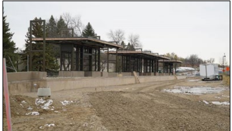
Opus Station construction underway in 2020
