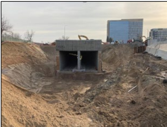
Hwy 62 LRT Tunnel- Halfway complete
