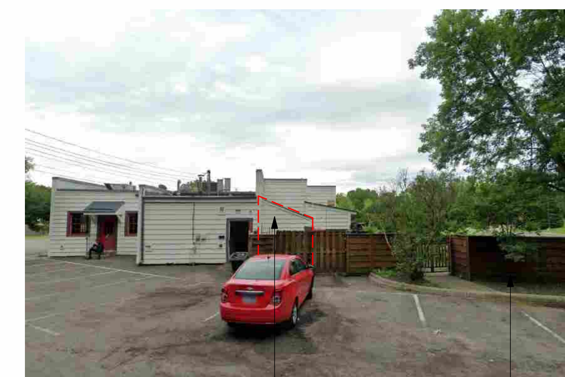
REMOVE EXIST OUTDOOR STORAGE LEAN-TO (6'-4" x 9'-4") FOR NEW EXTERIOR WALK-IN COOLER & WALK-IN FREEZER
