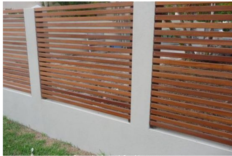
SEE-THROUGH FENCING AROUND POOL
