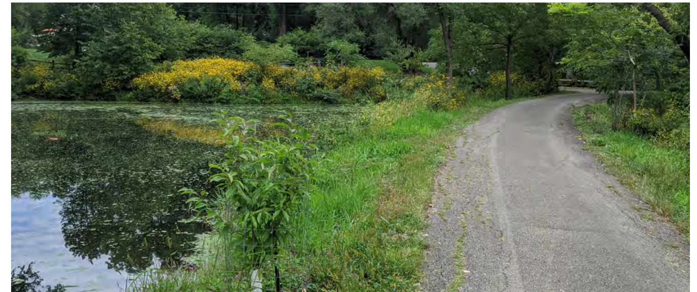
Above: A stormwater pond near the parking lot has a managed buffer of native species.
